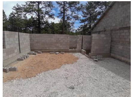
Construction in Natahuachi
